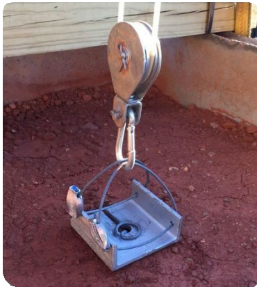
Twist anchor pullout test.
